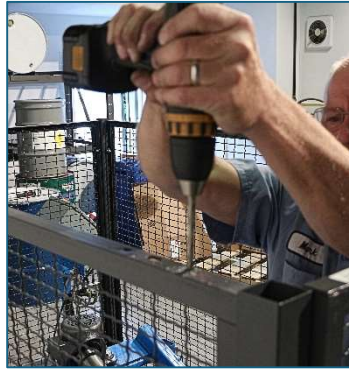
Drill holes for switch mounting plate.
