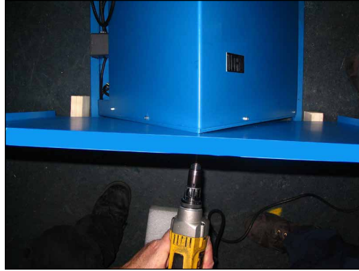
Step 7: Align each self drilling screw near the center of the angle frame.
